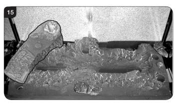
7.13 Place Log B on top of Log D. There is a hole on the underside of Log B which fits over the raised stud on Log D to secure in place. The right hand side of the log rests in the groove in the burner, see Diagram 16.
