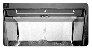
3.11 The baffle can now be removed through the front of the appliance.
